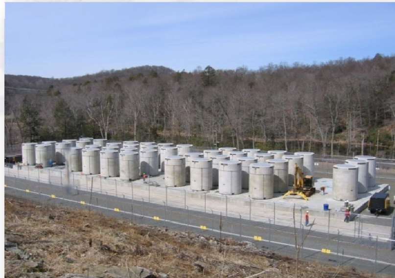
Dry cask storage for used fuel at the Surry station in Virginia
