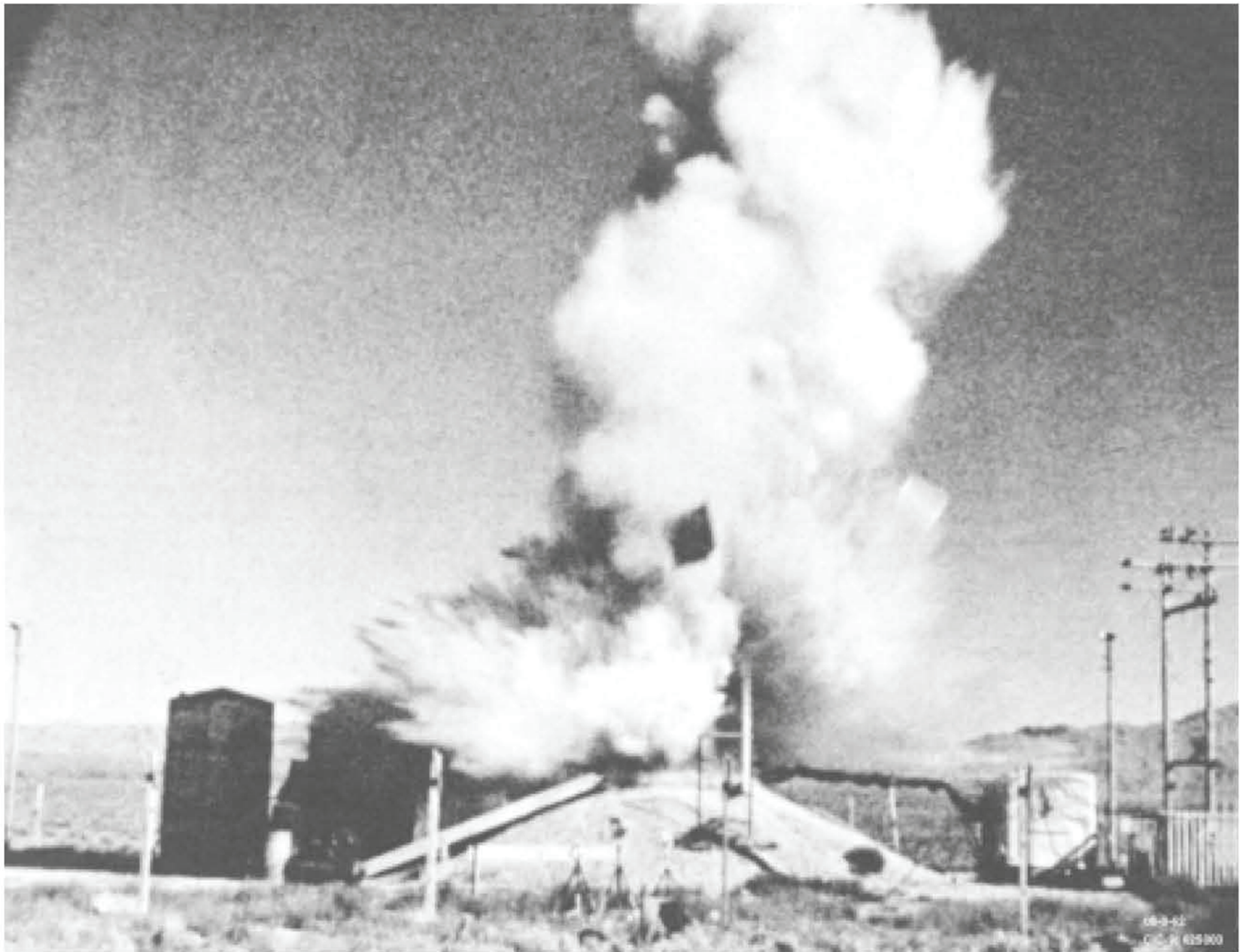
Figure 59. The destructive excursion in BORAX, 22 July 1954.
