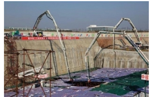
First Concrete poured for China's HTR-PM
