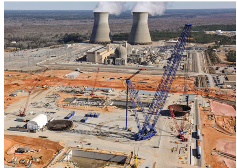
Vogtle 3 & 4, Courtesy of Georgia Power
