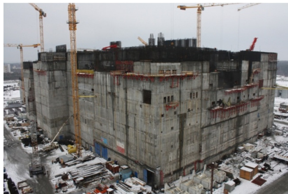
Reactor Compartment of Main Building
