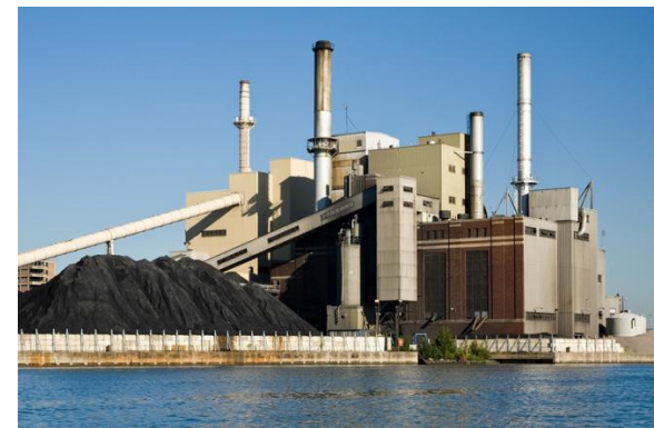
5 to 8 coal boilers
