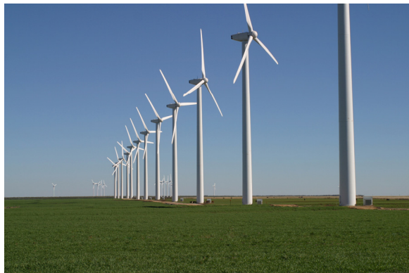
1670 to 2500 Wind Turbines (over 300 to 400 miles 2 )
