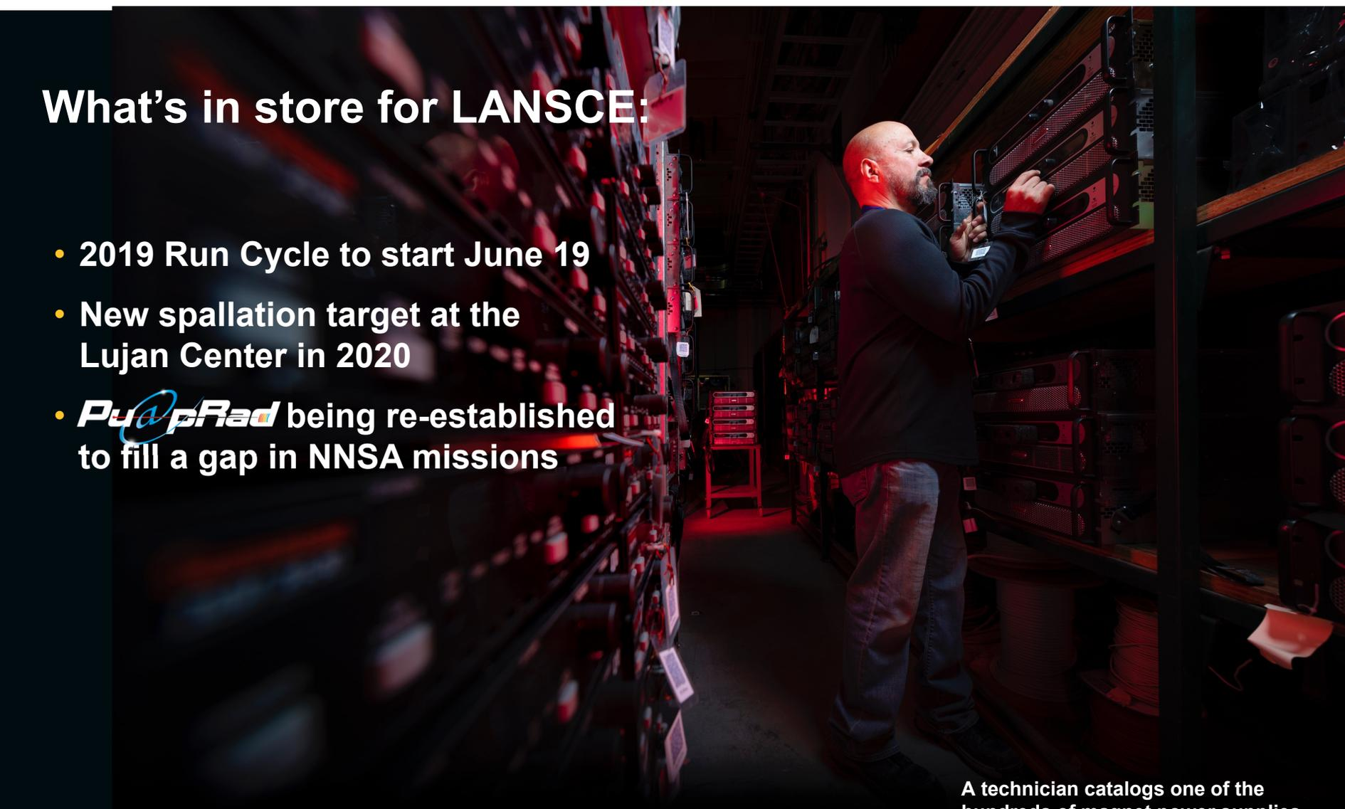
A technician catalogs one of the hundreds of magnet power supplies that keep the LANSCE accelerator operating efficiently.
