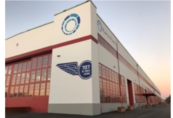
Kairos Power Headquarters
